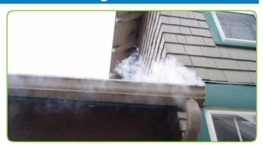
The City of Lansing is continuing efforts to repair the city's aging sanitary sewer system. In the next several weeks, customers may notice smoke coming from their sanitary sewers. This is part of a test to find leaks in the system. The non-toxic, odorless smoke is blownintosewermanholes, goesthrough the pipes, and comes out where there are broken pipes or where roof downspouts, outside area drains, or foundation drains are connected to the sanitary sewers.
