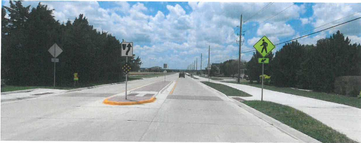
Figure 41 - Basic Raised Median with Pedestrian Refuge near Hall Street & W 41st Street in Hays, KS (Driver's Viewpoint)
