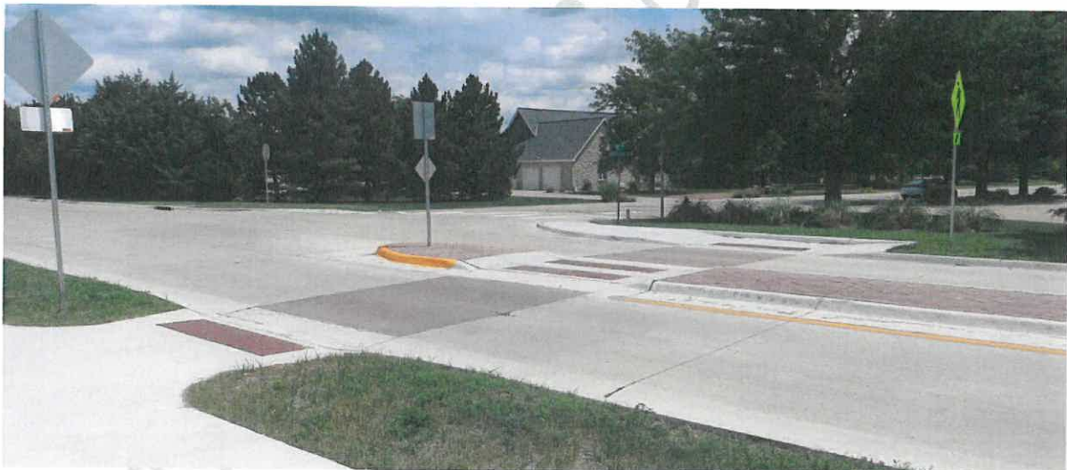
Figure 42 - Basic Raised Median with Pedestrian Refuge near Hall Street & W 41st Street in Hays, KS (from Sidewalk)
