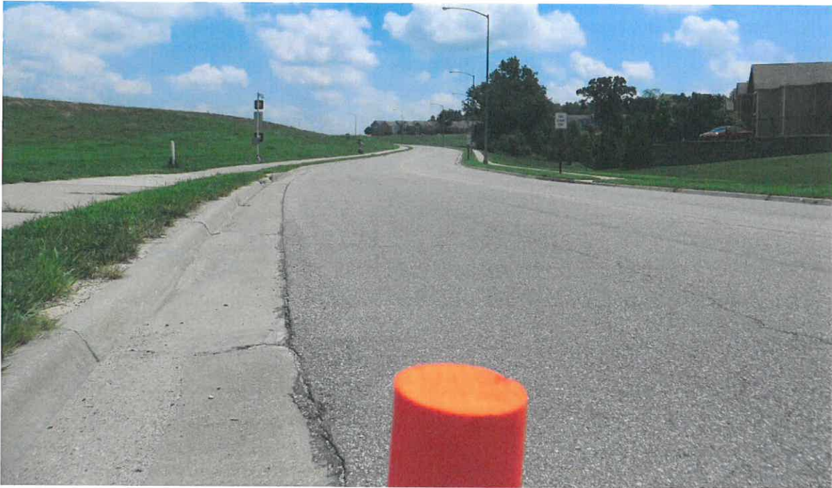
Figure 40 - Viewing Westbound Approach at Crosswalk Showing Sufficient Sight Distance to the East
