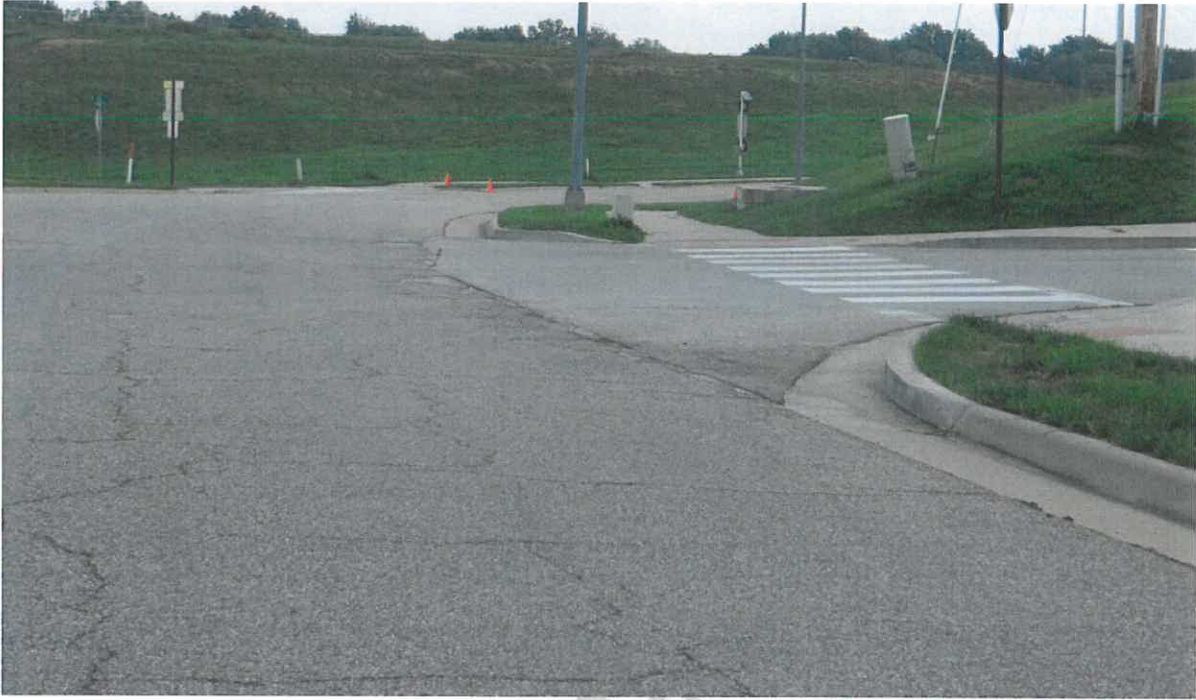
Figure 38 - Eastbound Approach with 2-Foot Object in View, 340 Feet Away (Moderate Zoom Photo)
